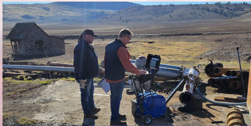
The well test found water at 200 feet and set the rebuilt pump at 350, offering good reliability for any future irrigation needs.
